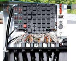
All the fuses and relays are grouped together in a centrally located box for easy access.
